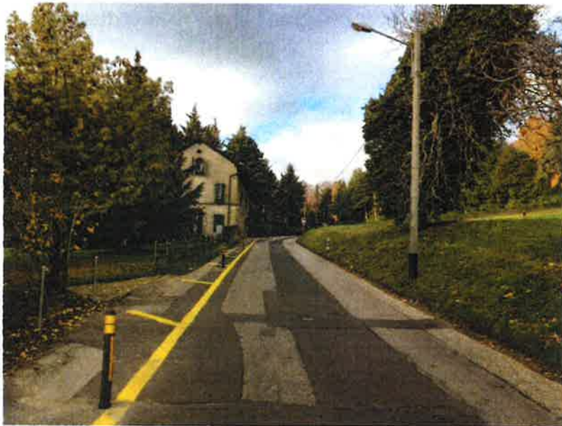
Figure 2 – Route de Champvent amont
